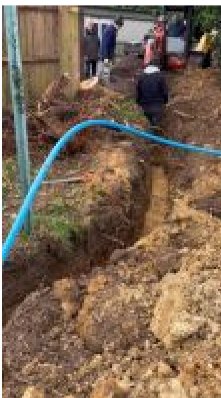
Trenching around conifer roots
