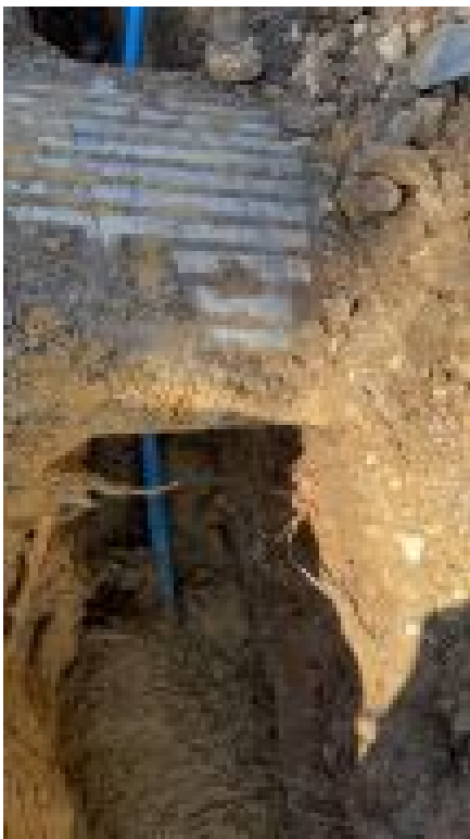
Trenching under speed hump
