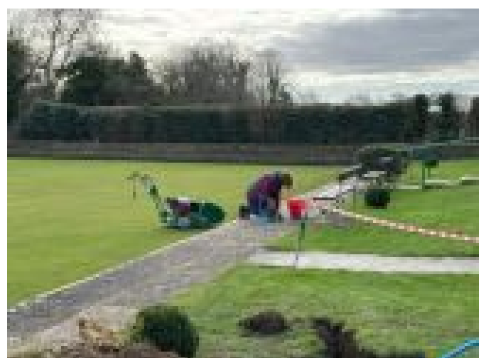
Weed removal from slabs
