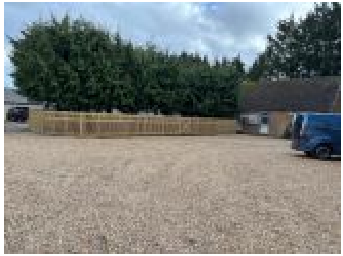
Flooding outside the Army Cadets hut corrected by spreading 20 tonne of flint.
