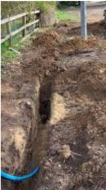
Hand dug trenching near street light
