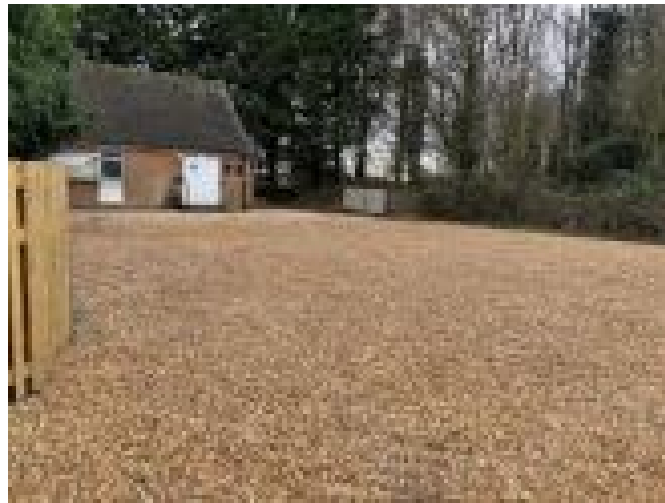
Flooding outside the Army Cadets hut corrected by spreading 20 tonne of flint.
