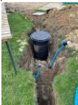
New water main stop tap chamber and upstand
